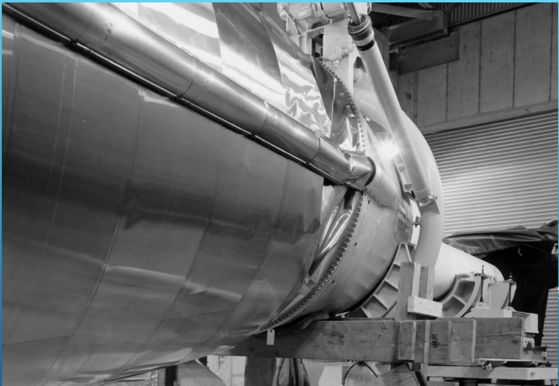
Atlas 69D (58-7064) * 549 th SMS LSB A-2 * Mead , NE 3000 PSI Helium line in Booster section ruptured causing LO2 Tank depressurization.
